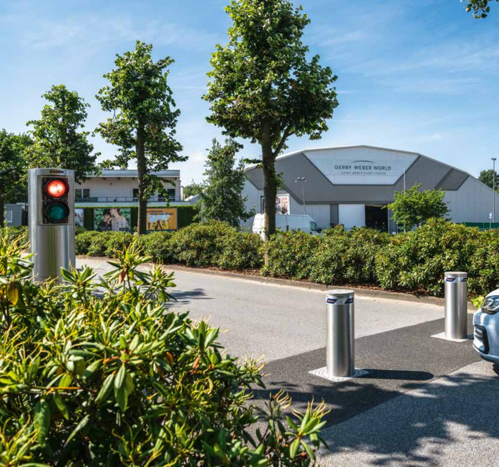
TOP LEFT. Automatic bollard with hydraulic operator
